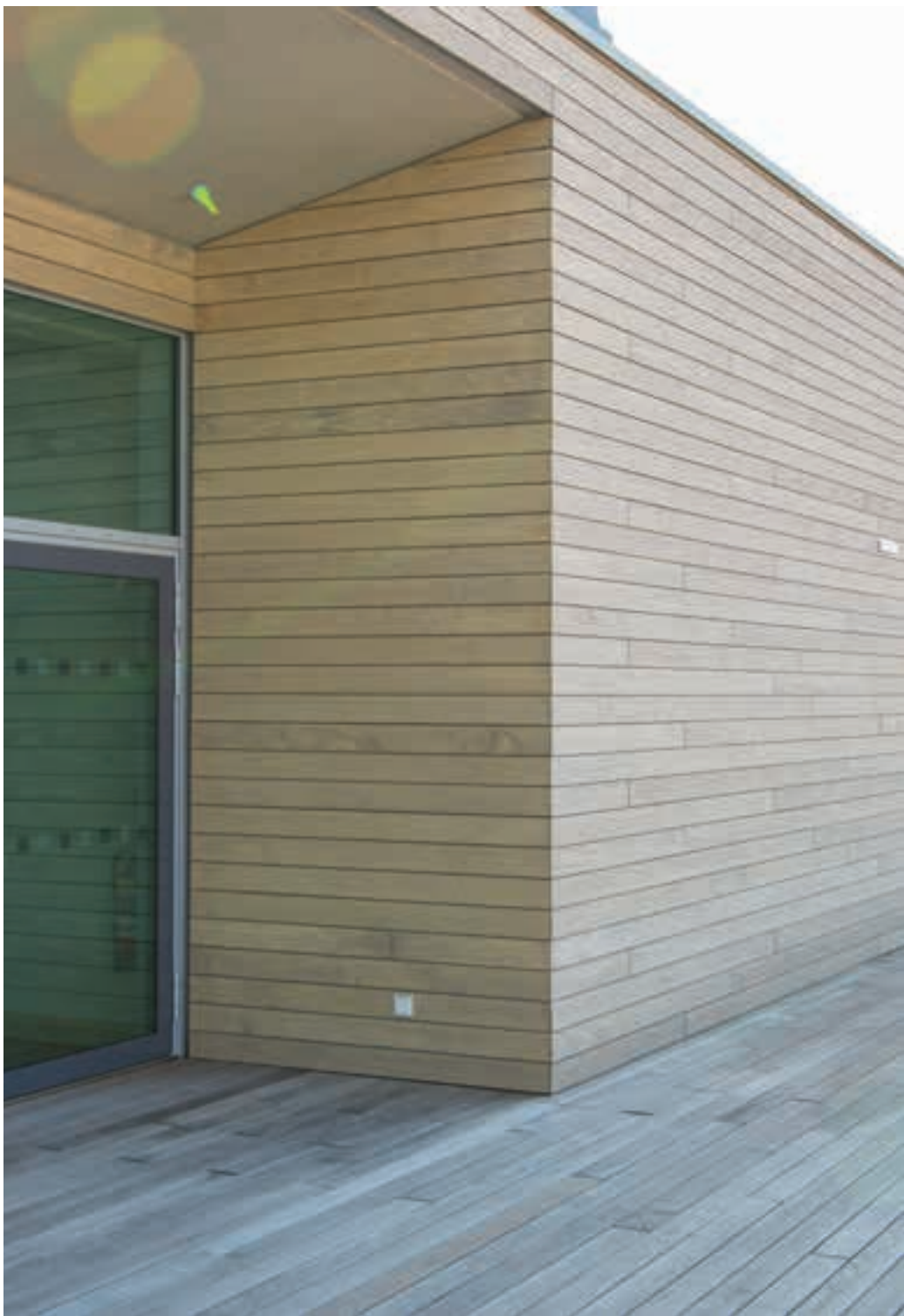
SCHOOL CENTER, ASPERN, AUSTRIA
