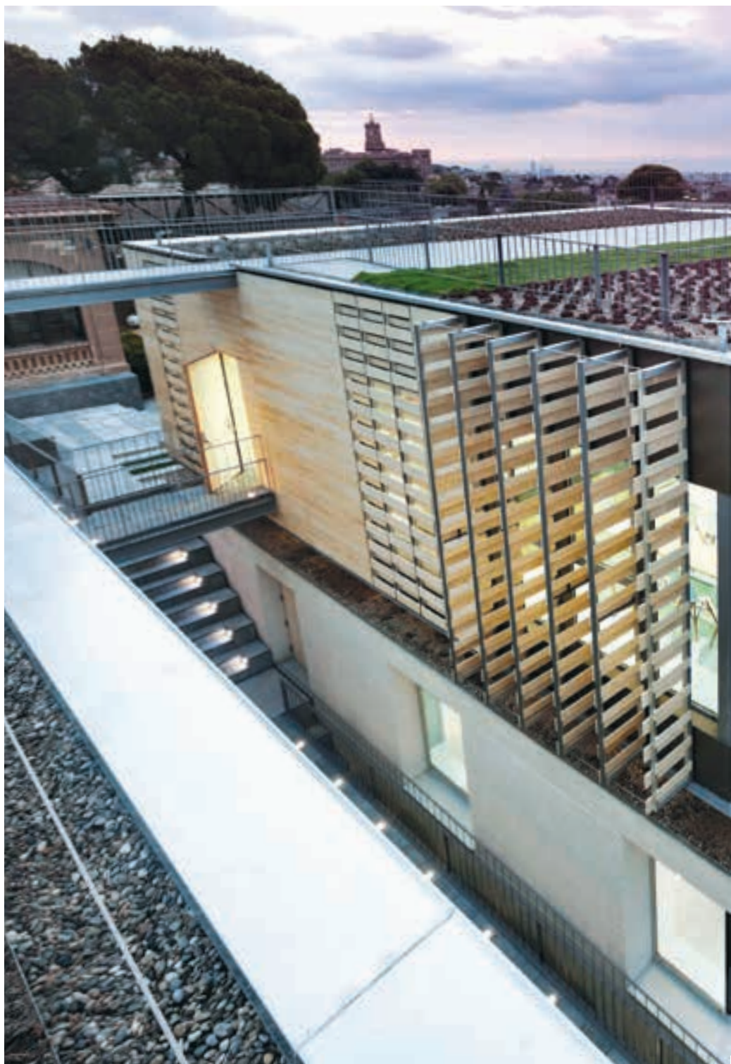
BACHILLERATO CAMPUS, BARCELONA, SPAIN
