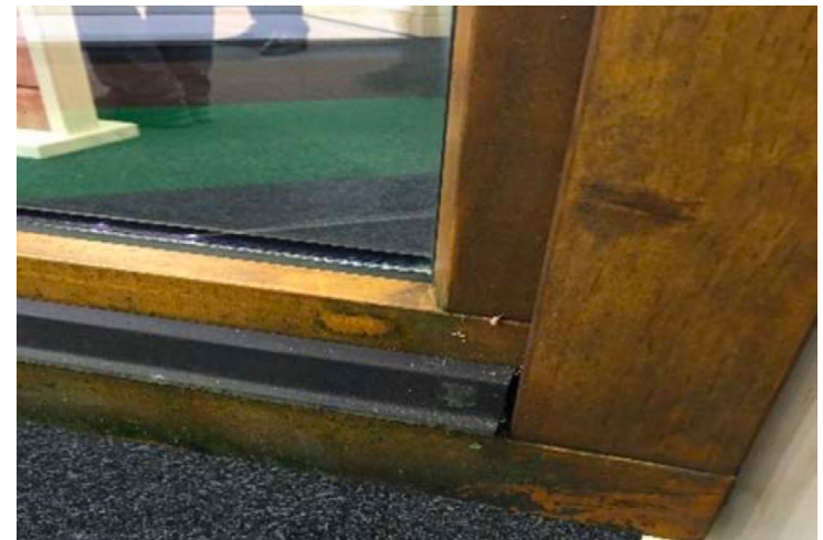
No coating degradation visible
